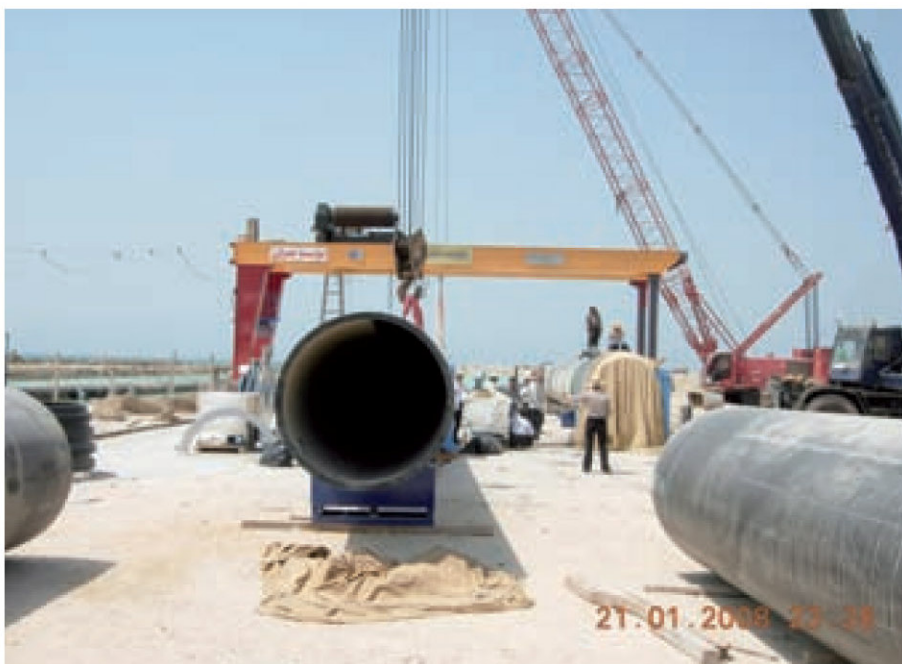
Fig. 12: Welding point with concrete paving slab and gantry crane. A pipe end is covered with a foil during welding to protect the heated tool from cooling and dust.
