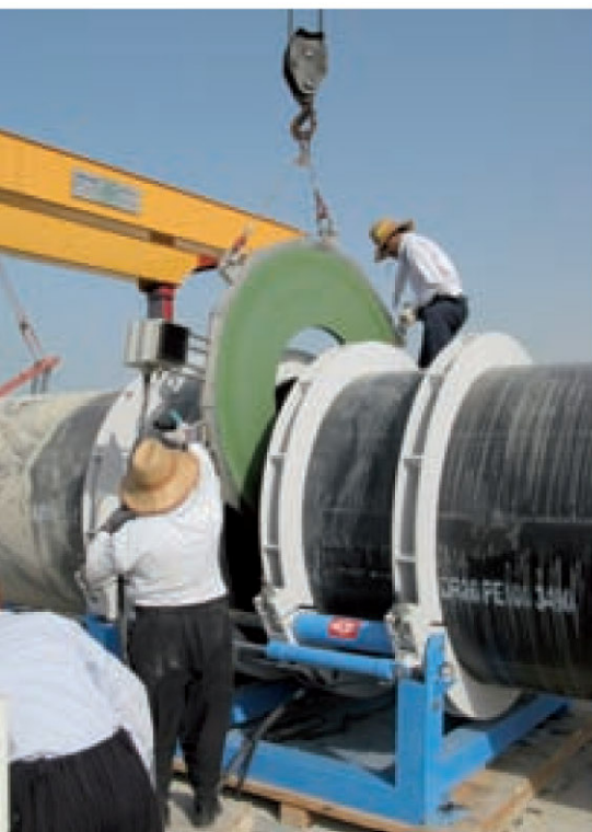
Fig. 13: Positioning of the heated tool by means of a crane
