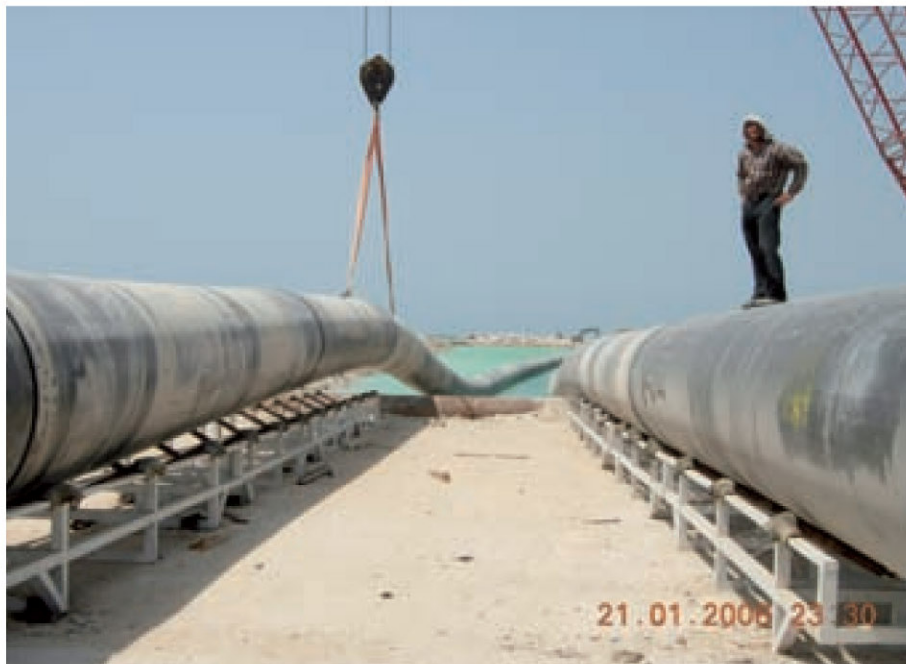
Fig. 11: Storage and pushing forward of the pipelines on pulley blocks
