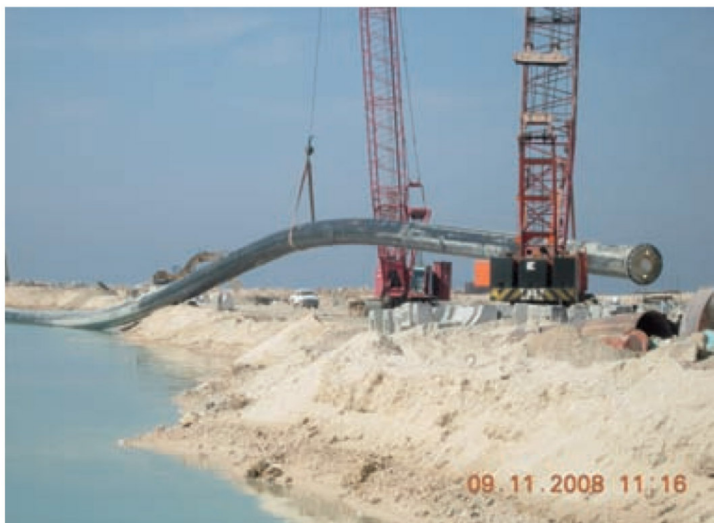
Fig. 10: Sealed PE pipeline is lifted into the dock by a crane
