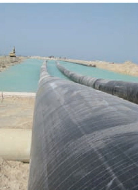
Fig. 9: Artificial dock for the interim storage of the 250 m long pipelines
